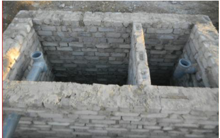
A two-chamber septic tank under construction.
