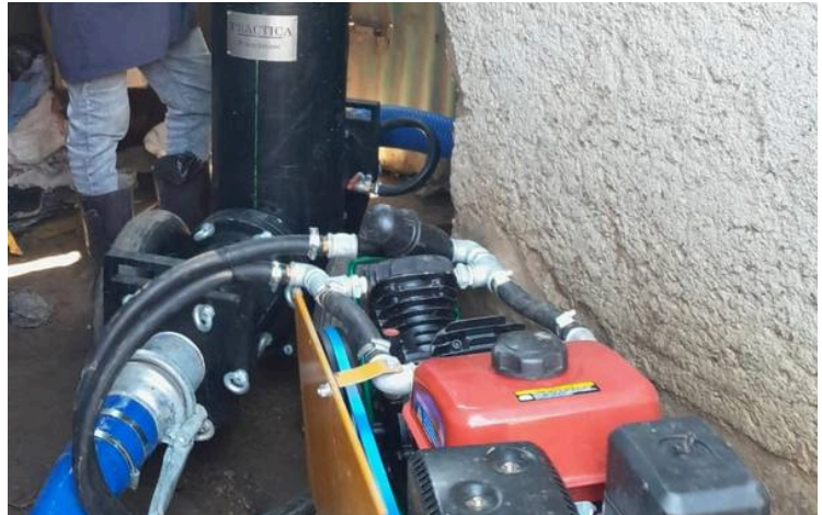
A trained operator emptying a pit with a PuPu pump.
